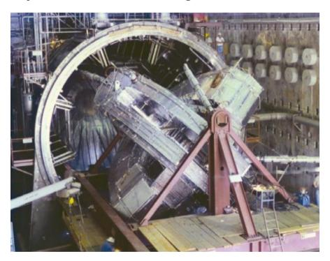
LLNL The MFTF under construction in 1981. The reactor was fully completed, but then mothballed before it could ever run an experiment! The reactor vessel and structures weigh 8 million pounds, including 3 million pounds of superconducting magnets, designed to confine a plasma at more than 100 million degrees.
